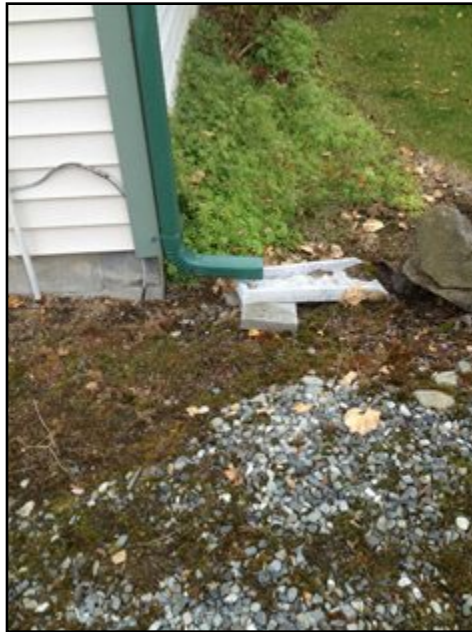
Downspouts end too close to building
