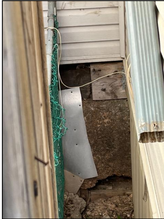
8. Siding - incomplete / missing
