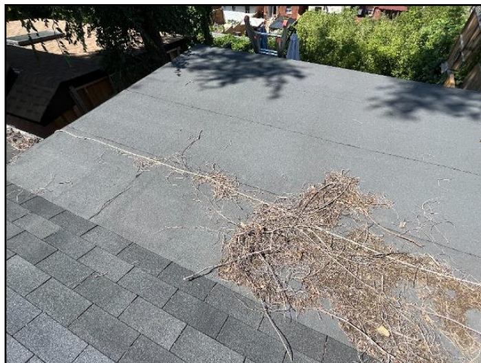
2. Modified bitumen membrane
