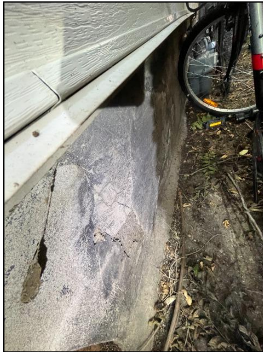
18. Parging damaged or missing
