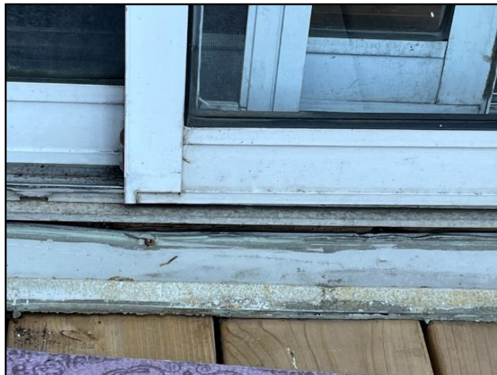
14. Sill deteriorated
