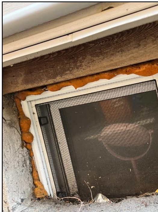
12. Flashing loose, missing or deteriorated
