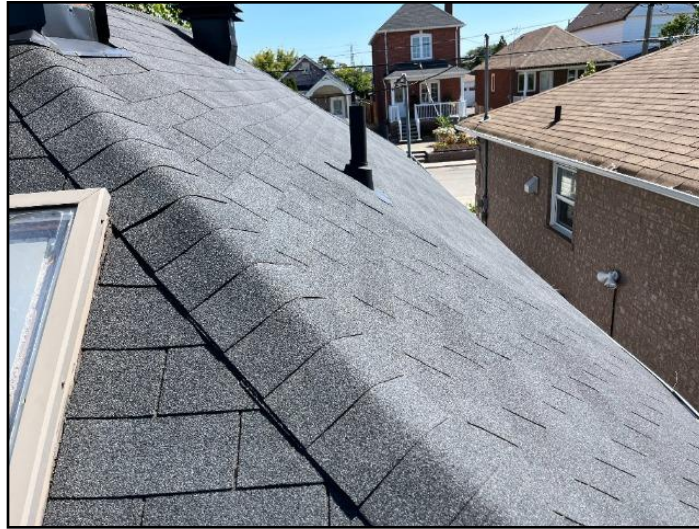
1. Asphalt shingles
