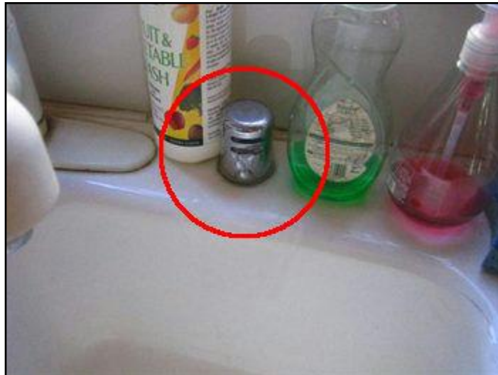
16. Backflow prevention defective
