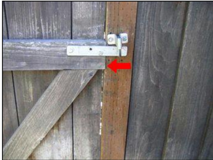
7. Gate - adjustment needed
