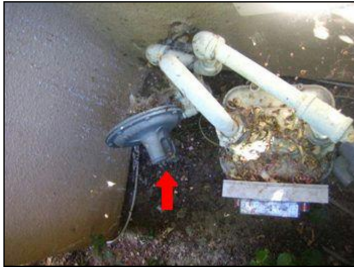
13. No wrench for gas meter shutoff valve
