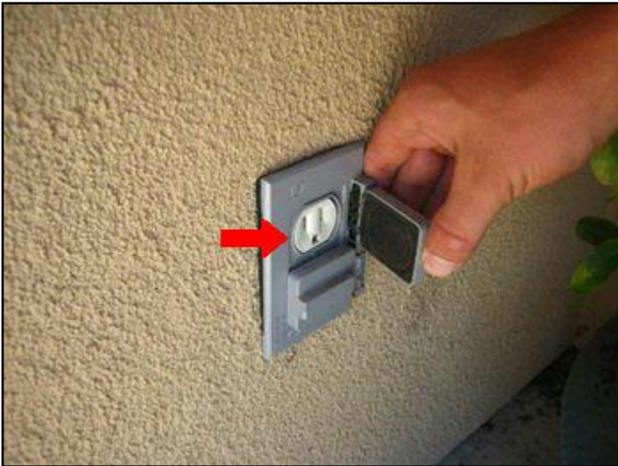
10. No GFCI apparent-Exterior
