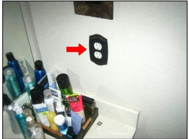
11. No GFCI apparent-Bathroom
