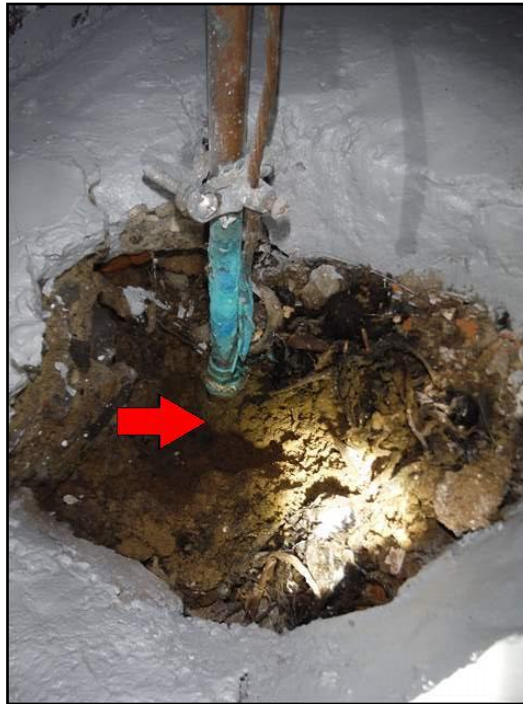
Obsolete Piping (Lead/Galv)
