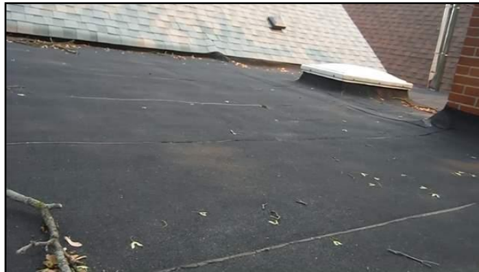
Modified bitumen membrane
