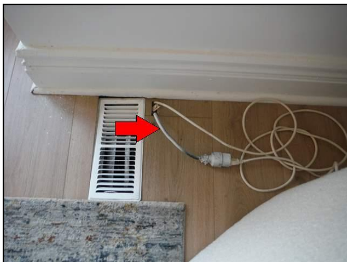
Extension cord used as permanent wiring
