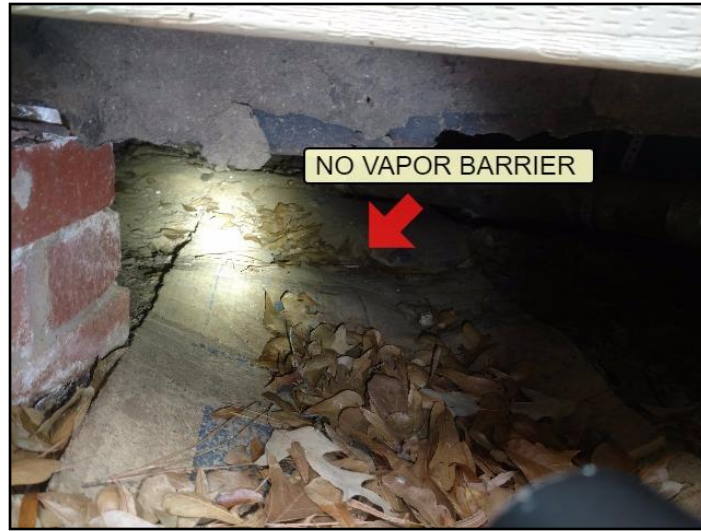
12. No vapor barrier in the crawl space...
