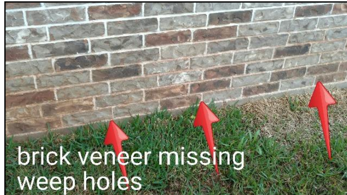
7. Missing, ineffective weep holes or flashings
