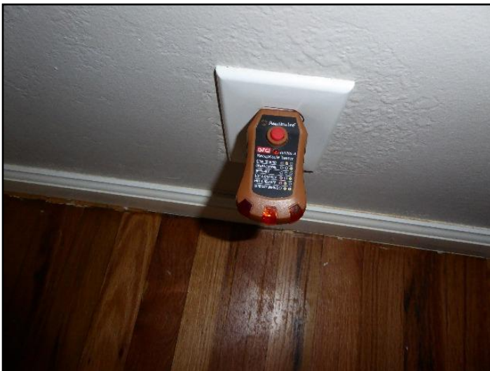
34. Ground needed for 3-slot outlet
