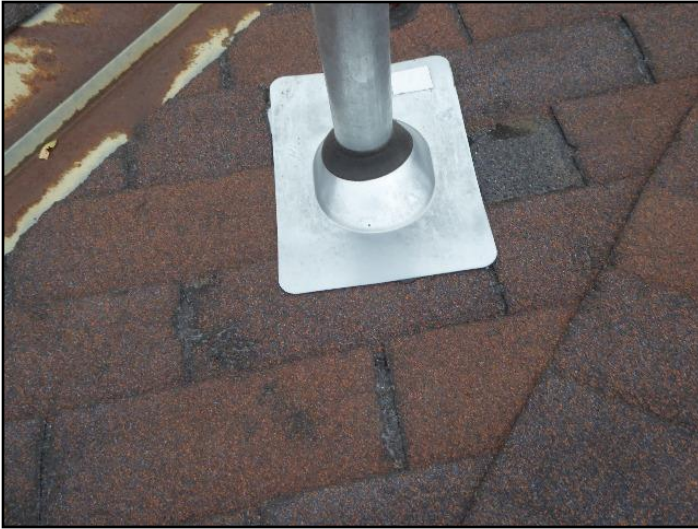
10. Improper flashing installation
