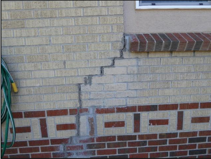
17. Settling cracks
