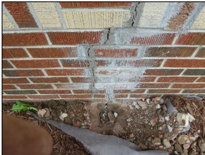
25. Settling cracks
