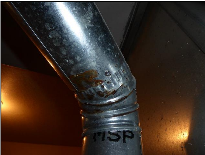
46. Poor connections
