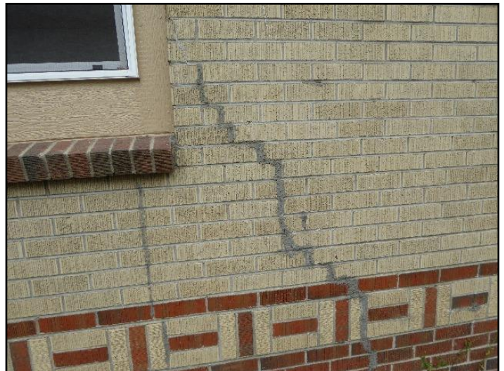
24. Settling cracks
