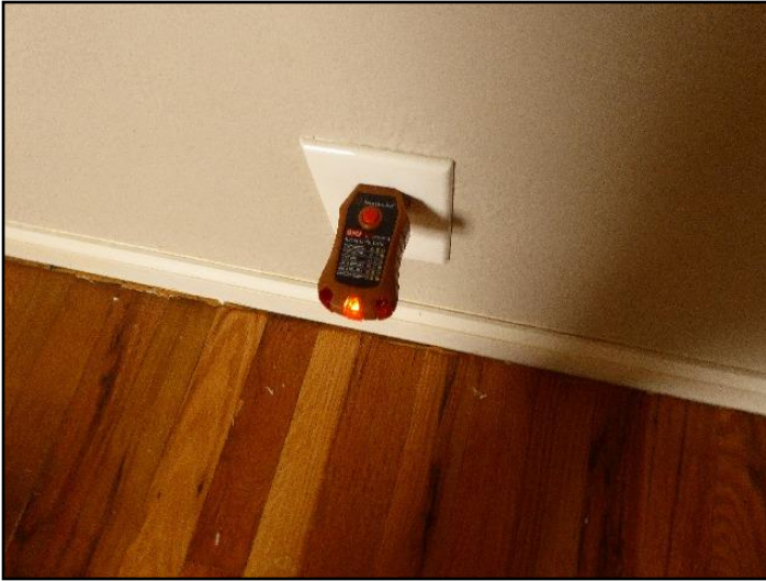
36. Ground needed for 3-slot outlet
