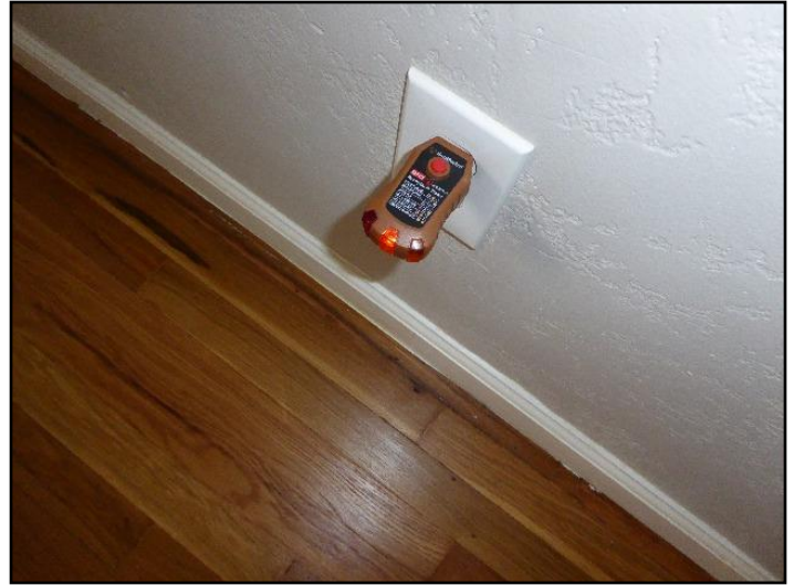
37. Ground needed for 3-slot outlet
