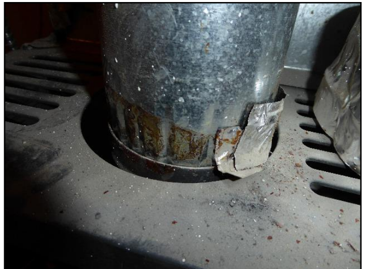
47. Poor connections
