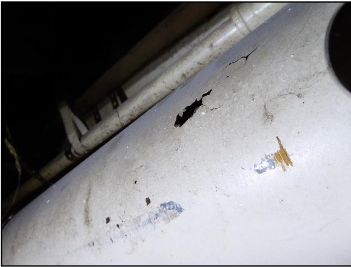
44. Safety issue. Rust holes in furnace vent pipe
