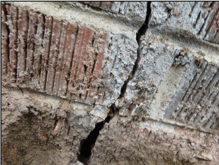
19. Cracks below grade
