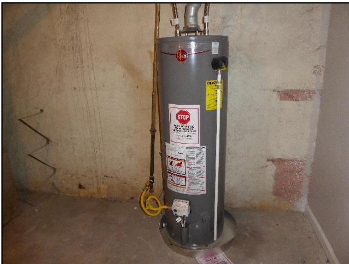
50. No floor drain for water heater
