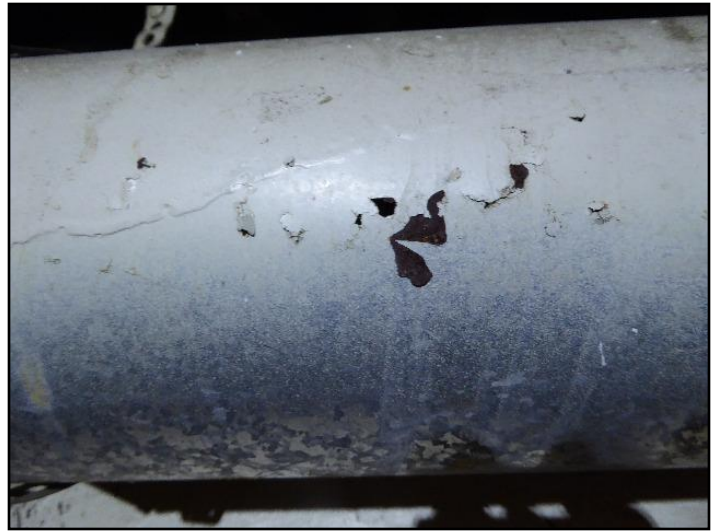
45. Safety issue. Rust holes in furnace vent pipe
