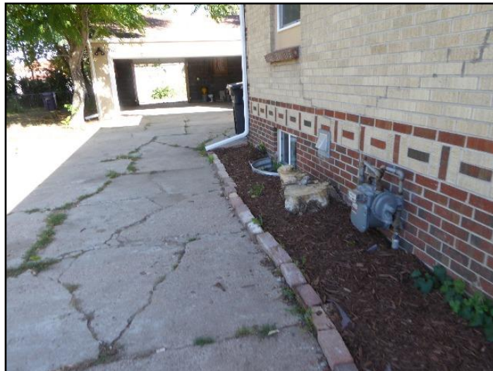
28. Cracked or damaged surfaces
