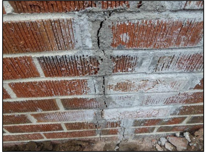
22. Settling cracks
