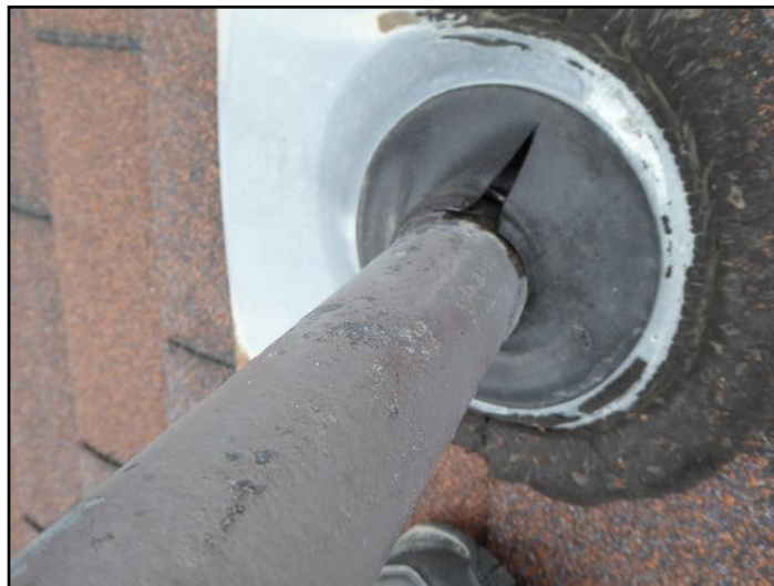
12. Cracked boot seal
