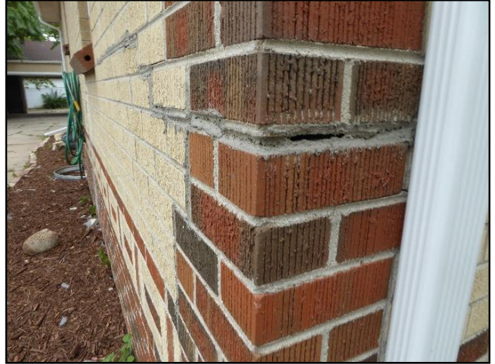
18. Settling cracks
