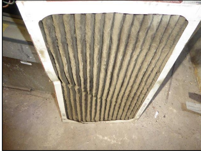
41. Furnace filter is clogged
