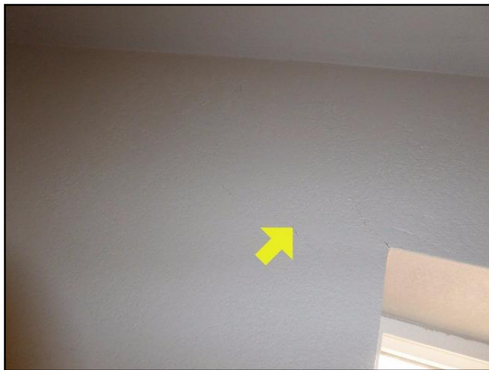
30. Settling cracks in drywall
