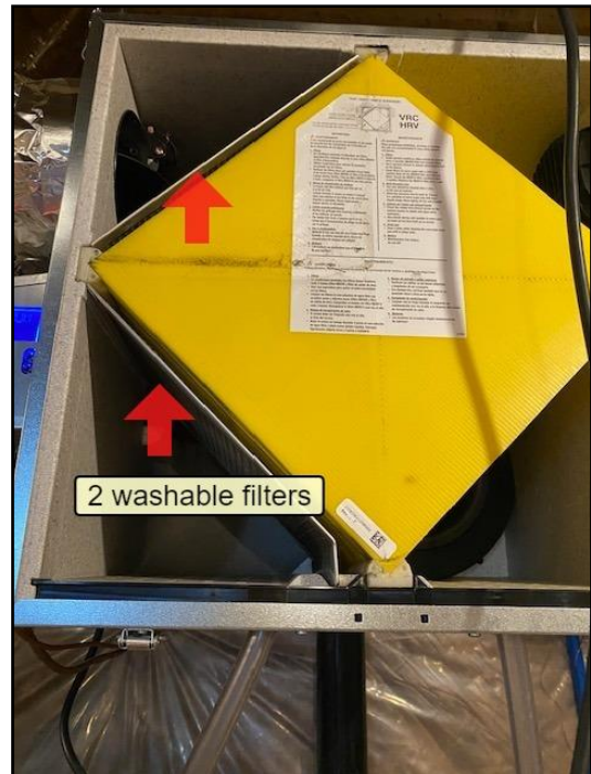
15. Heat recovery ventilator (HRV)
