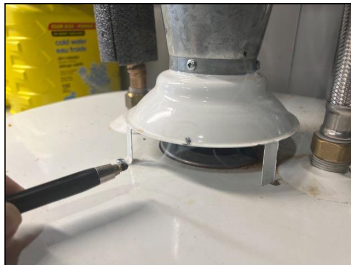
14. House Depressurization (Non Conforming)
