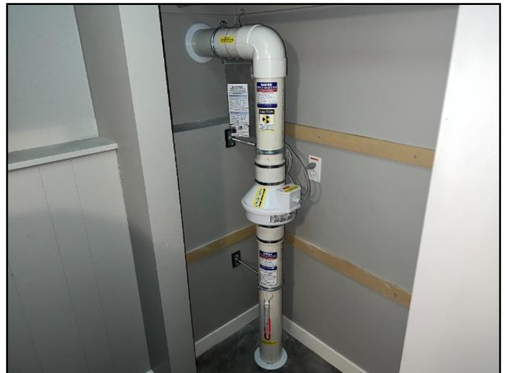
10. Radon mitigation completed system pictures
