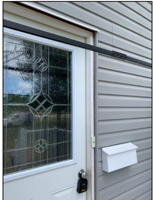
39. Flashings missing
