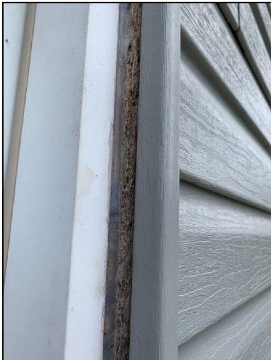
38. Flashings missing
