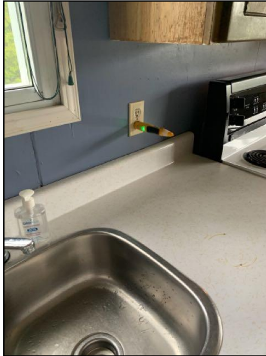
97. GFCI/GFI needed (Ground Fault Circuit...
