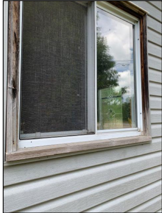
73. Paint or aluminum cap window frames. Seal...
