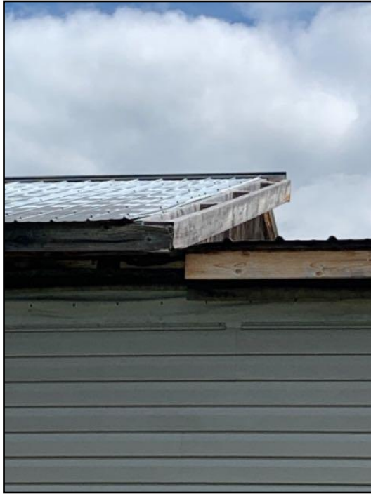
10. Missing, loose or broken pieces
