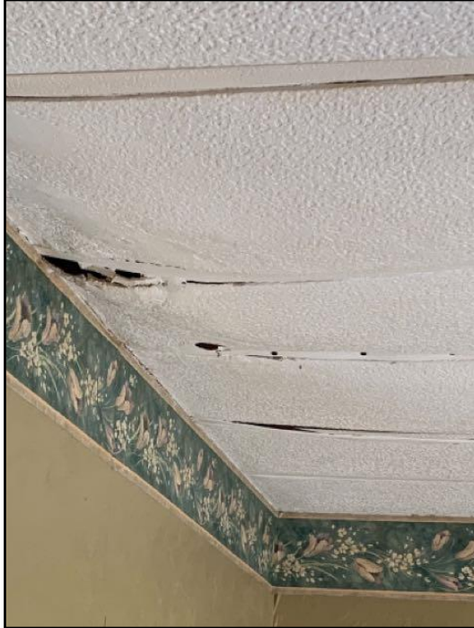
162. Water damage
