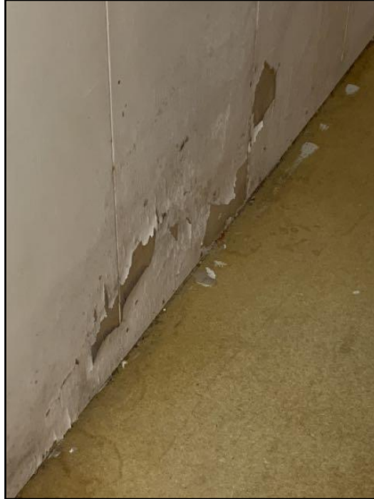
167. Water damage
