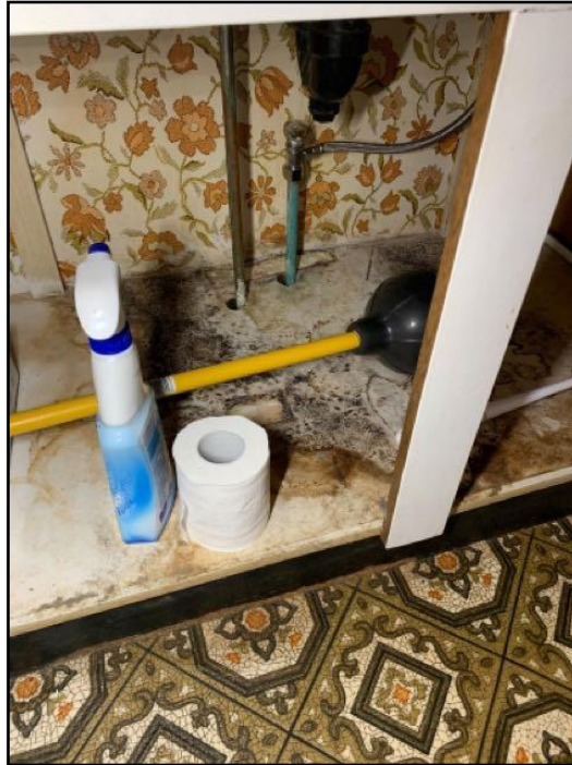
189. Water damage
