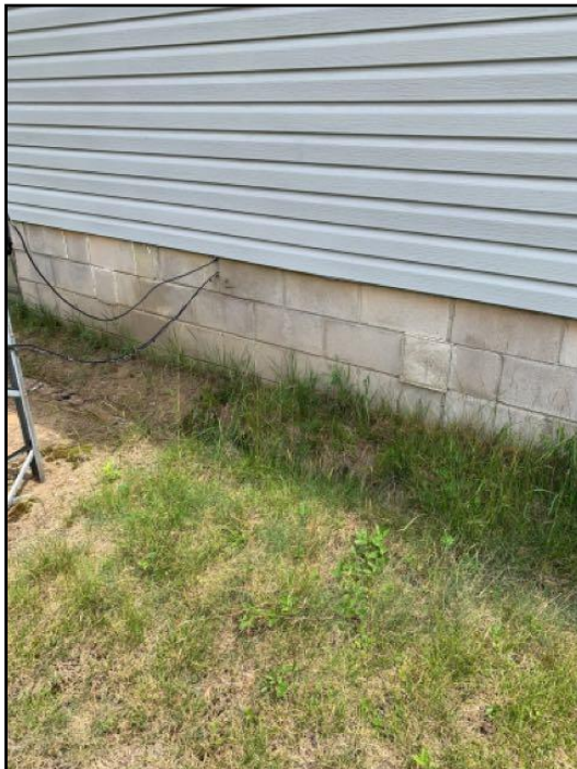
69. Parging damaged or missing
