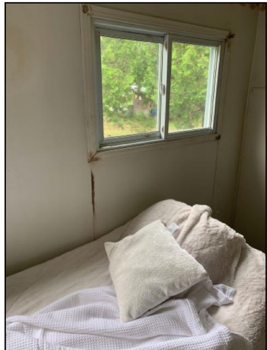
166. Water damage
