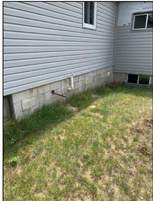
70. Parging damaged or missing
