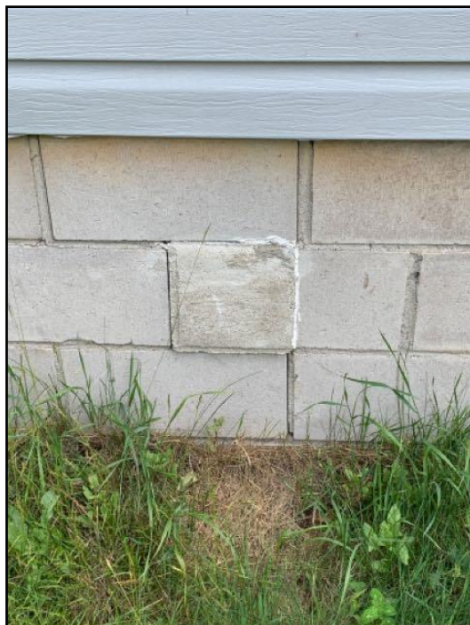
65. Mortar deterioration
