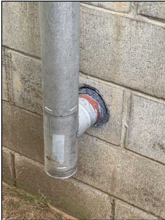
43. Caulking missing or ineffective
