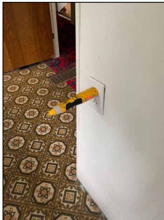
95. Reversed polarity
