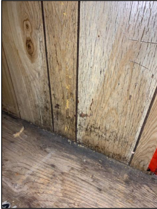
168. Water damage
