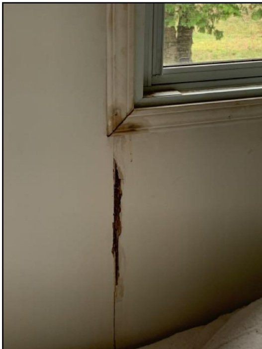
165. Water damage
