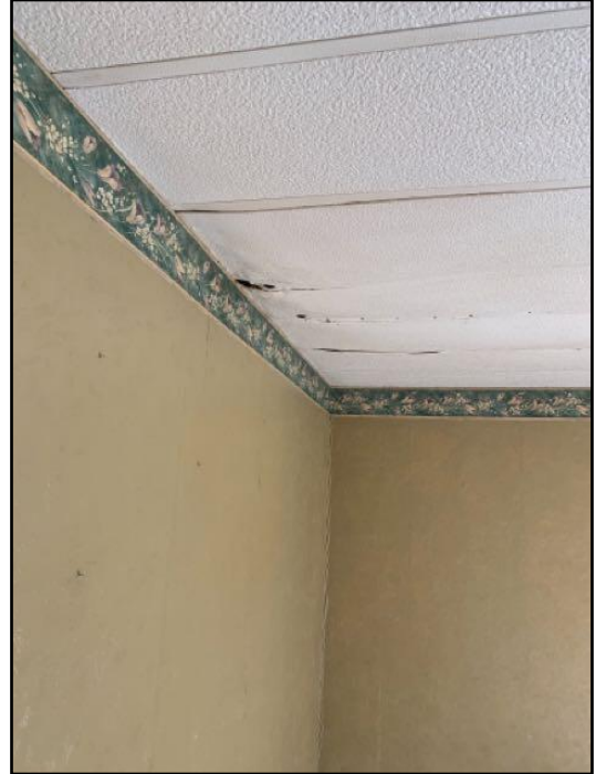
163. Water damage
