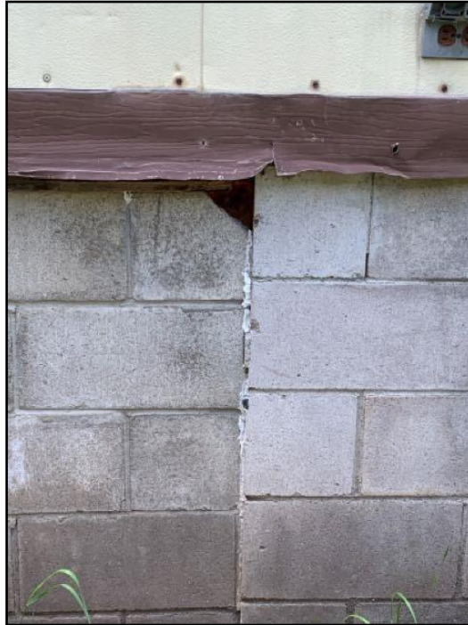
40. Caulking missing or ineffective
