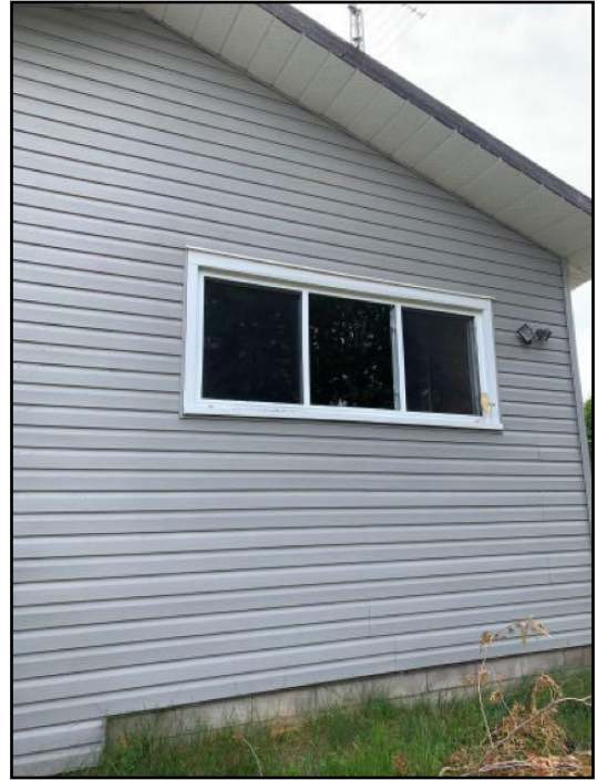
42. Caulking missing or ineffective
