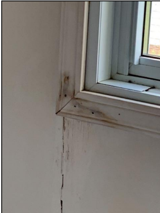
190. Water damage
