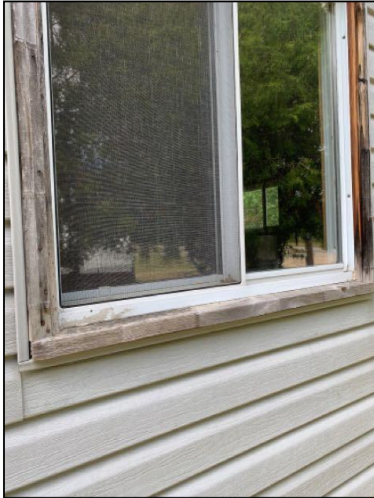
72. Paint or aluminum cap window frames. Seal...
