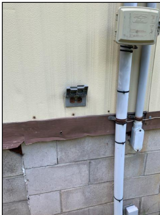
96. GFCI/GFI needed (Ground Fault Circuit...
