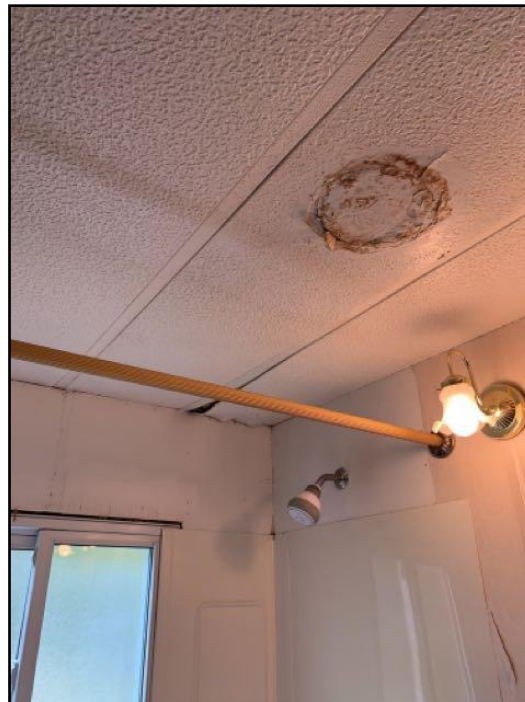
161. Water damage
