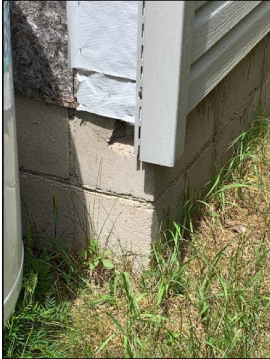
63. Masonry deterioration
