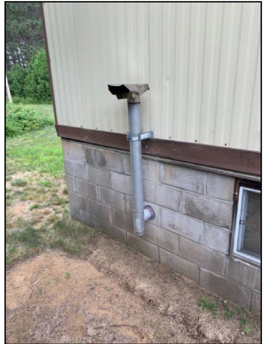
44. Caulking missing or ineffective
