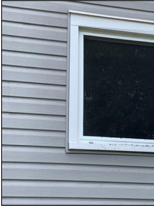
41. Caulking missing or ineffective
