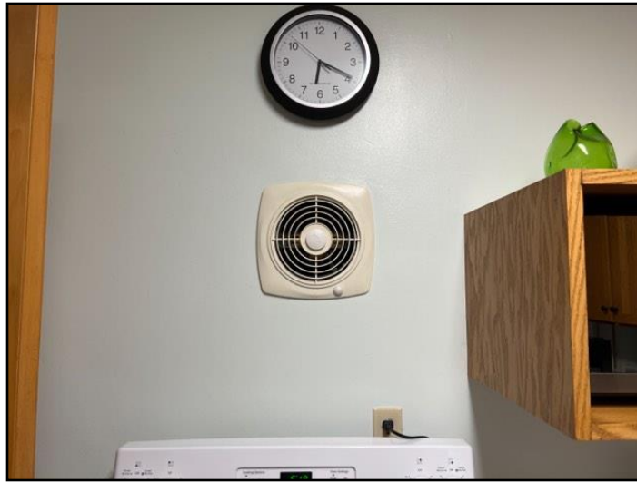
103. Exhaust fan discharges to the exterior
