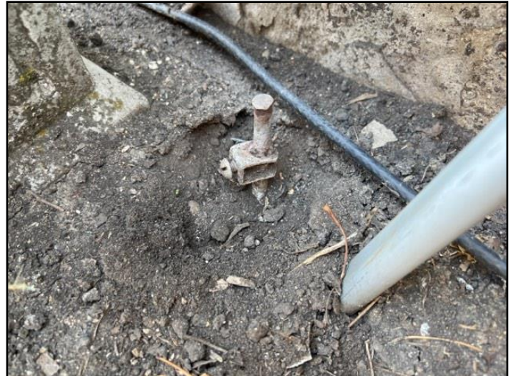
55. Copper - ground rods
