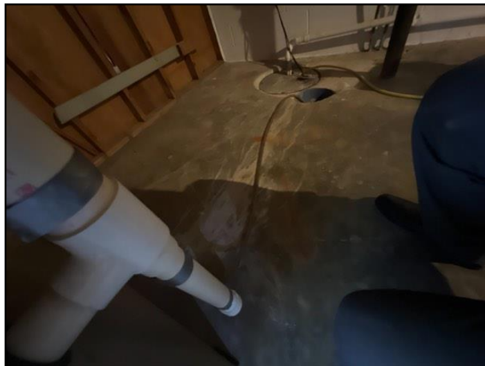
68. Discharges into floor drain
