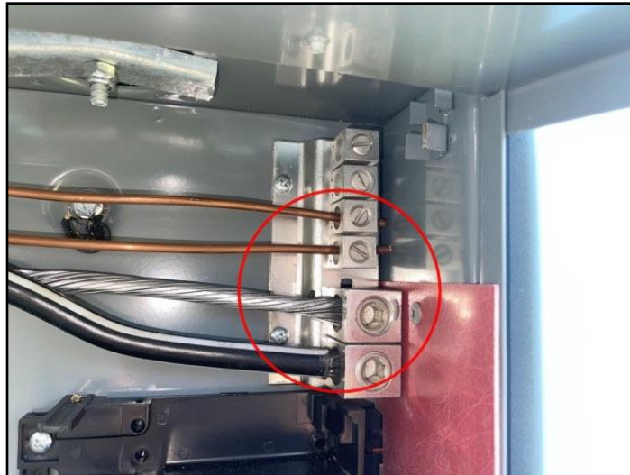
Neutral and ground bonded at service.
