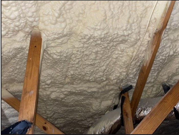
Sprayed foam attic insulation.
