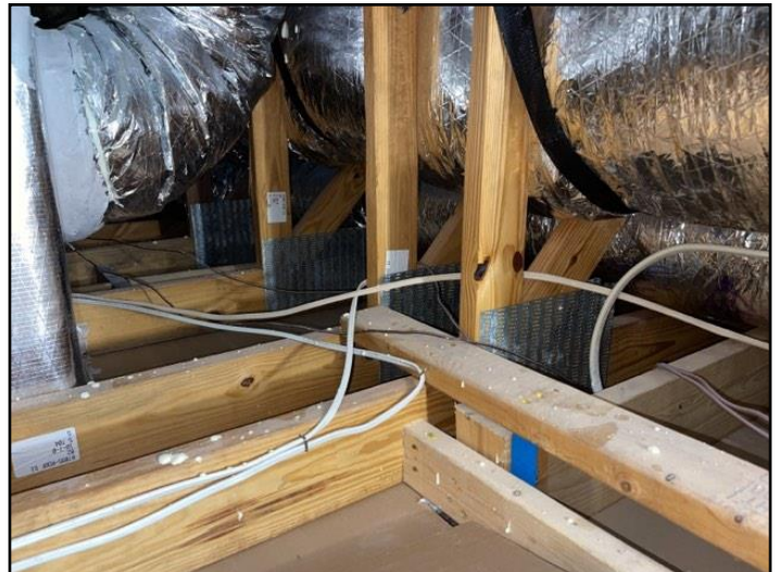
Engineered roof trusses.
