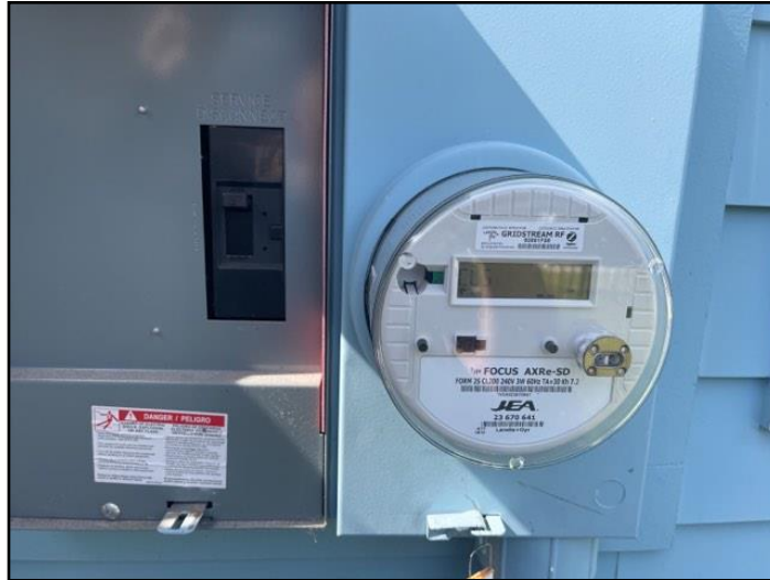
150 Amps (240 Volts) meter and disconnect.
