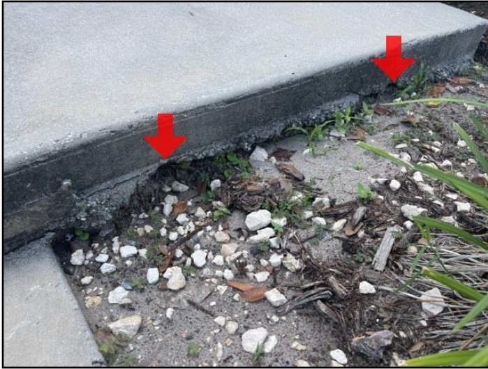
Minor erosion at front steps stoop.
