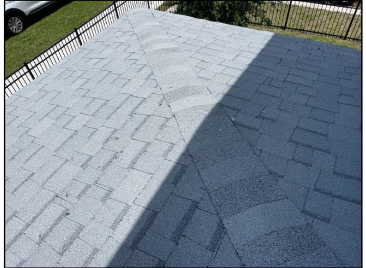
Architectural fiberglass/asphalt shingles.
