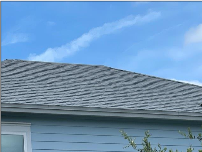
Architectural fiberglass/asphalt shingles.
