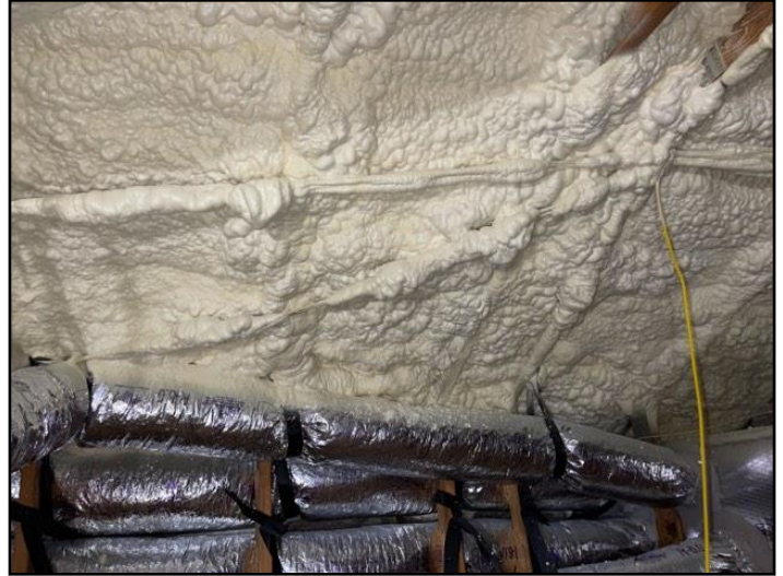
Sprayed foam attic insulation.
