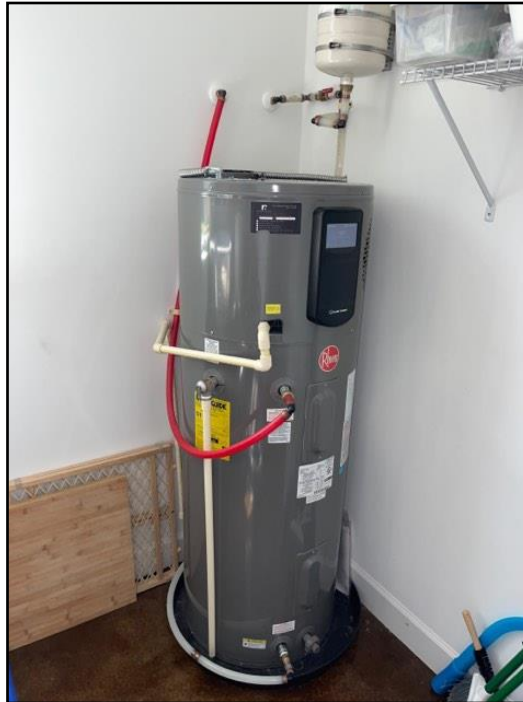
Rheem high efficiency heat pump water heater.
