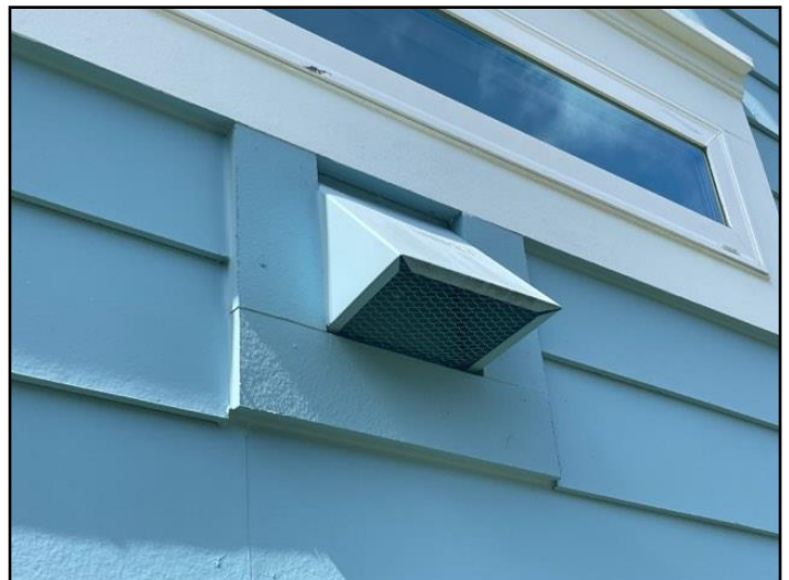
Microwave range fan vented to the exterior
