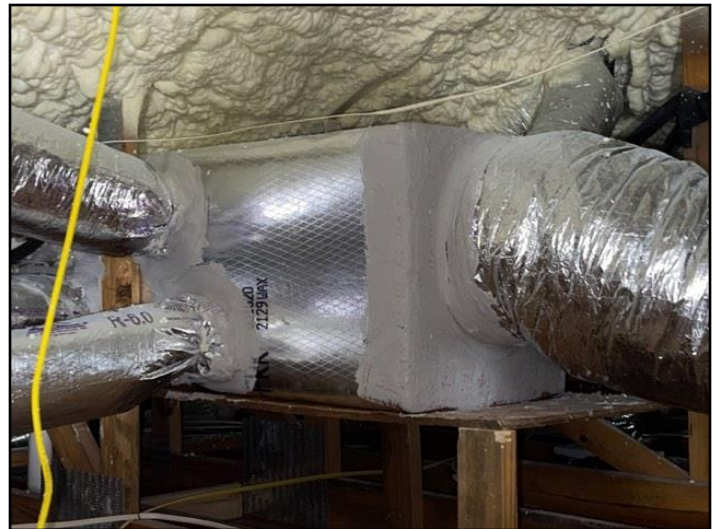
Foam board and flex ducts.
