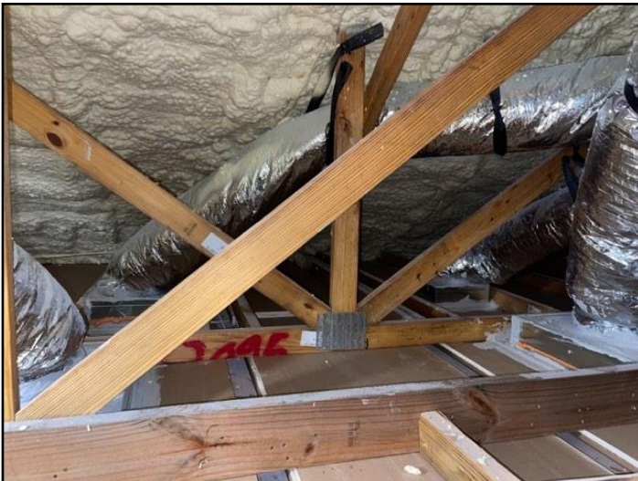
Engineered roof trusses.
