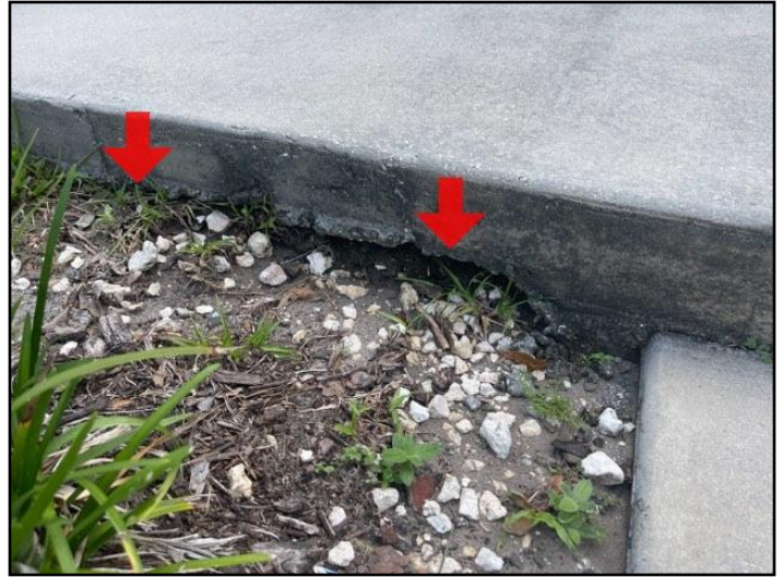
Minor erosion at front steps stoop.
