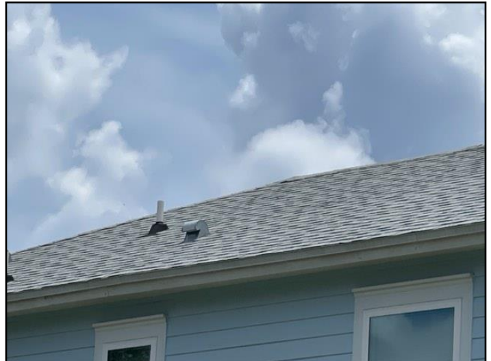
Architectural fiberglass/asphalt shingles.
