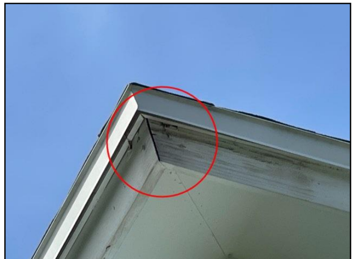
Rot starting at left-rear fascia corner.
