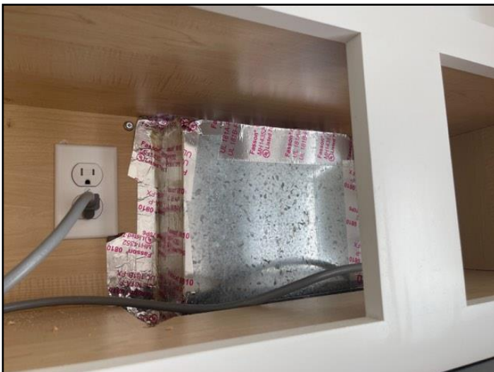
Microwave range fan vented to the exterior
