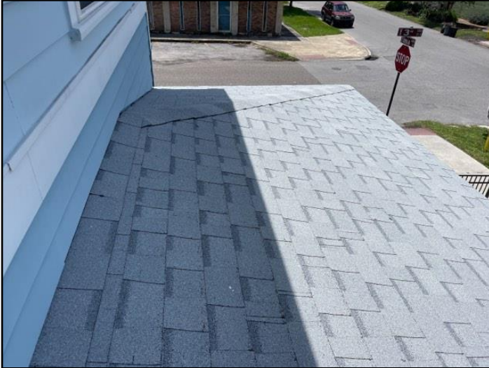
Architectural fiberglass/asphalt shingles.
